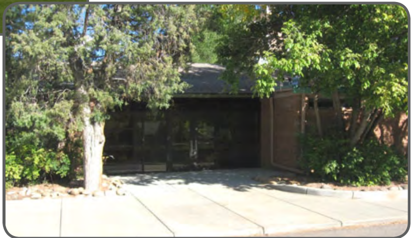
Modified ADA entrance to Lyons Elementary School
