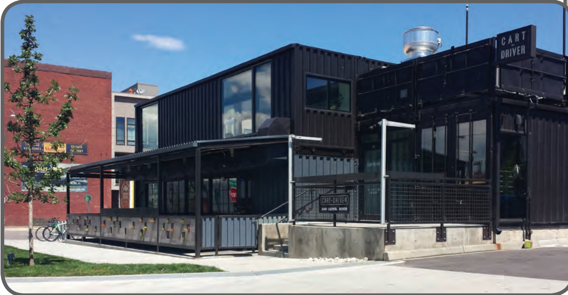
25th & Larimer - Shipping Container Project, Denver, Colorado
